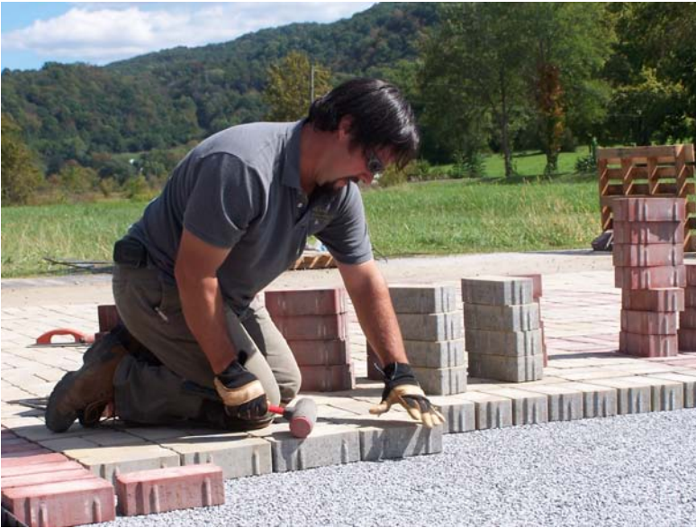
Chad Owens of Owens Landscaping of Abingdon installed the permeable pavers in the parking lot at Saltville. Above, the completed handicapped spaces located at the trail head.
