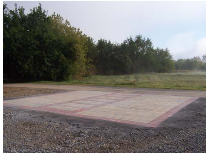
Chad Owens of Owens Landscaping of Abingdon installed the permeable pavers in the parking lot at Saltville. Above, the completed handicapped spaces located at the trail head.
