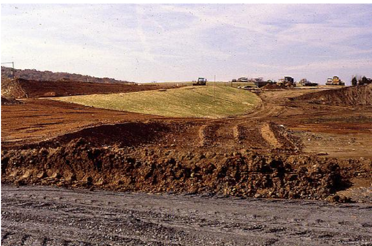
Land disturbing activity with erosion control measures in place.
