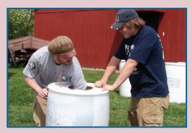
measure about one inch above bottom of barrel where barrel begins to rise toward top. Using a 3/4 inch spade bit, drill a hole through the barrel side.
